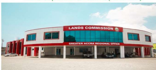
Phase II Under Construction
