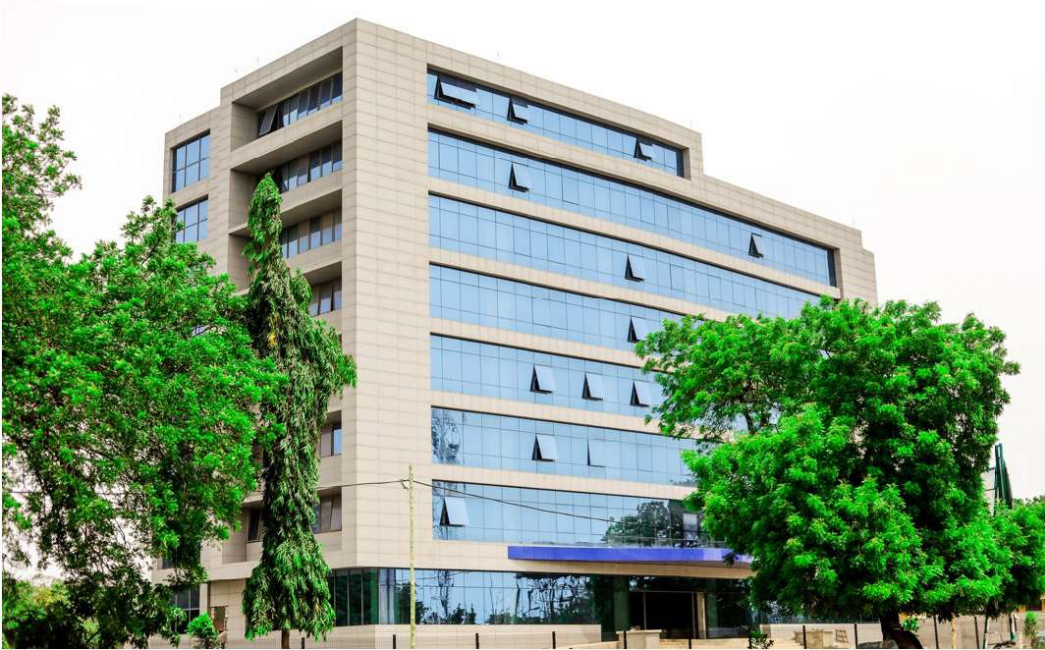
Figure 4: Construction of New Corporate Head Office Building
