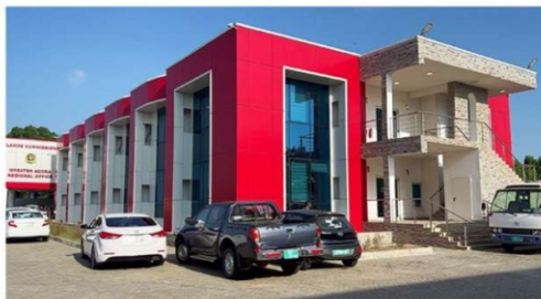
Completed Phase I
